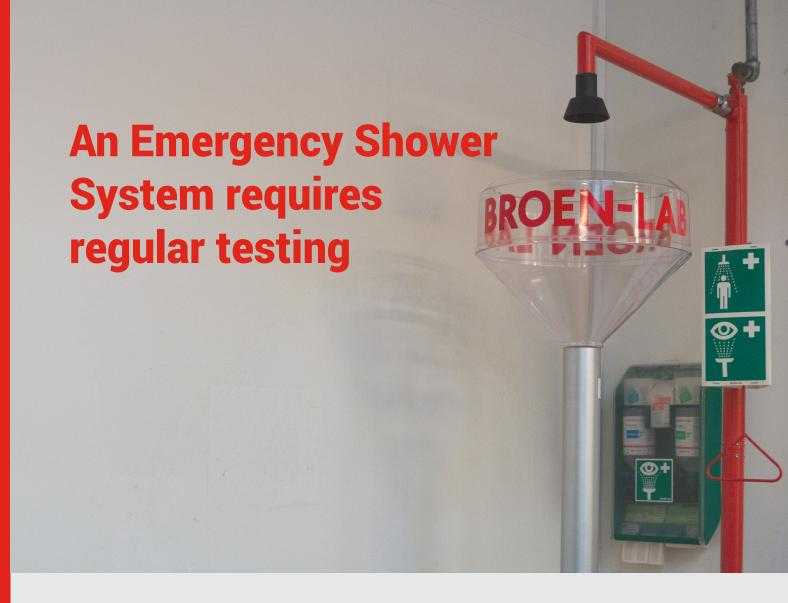
To secure the safety of your employees, both European and American standards recommend that you test your Emergency Shower System regularly. With the specially designed test equipment from BROEN-LAB the testing of water volume, flow rate, and spray pattern can be carried out quickly and hygienically by just one person.
